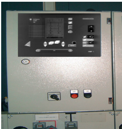
Fig. 3 Display and operating unit, integrated in the medium voltage cell
